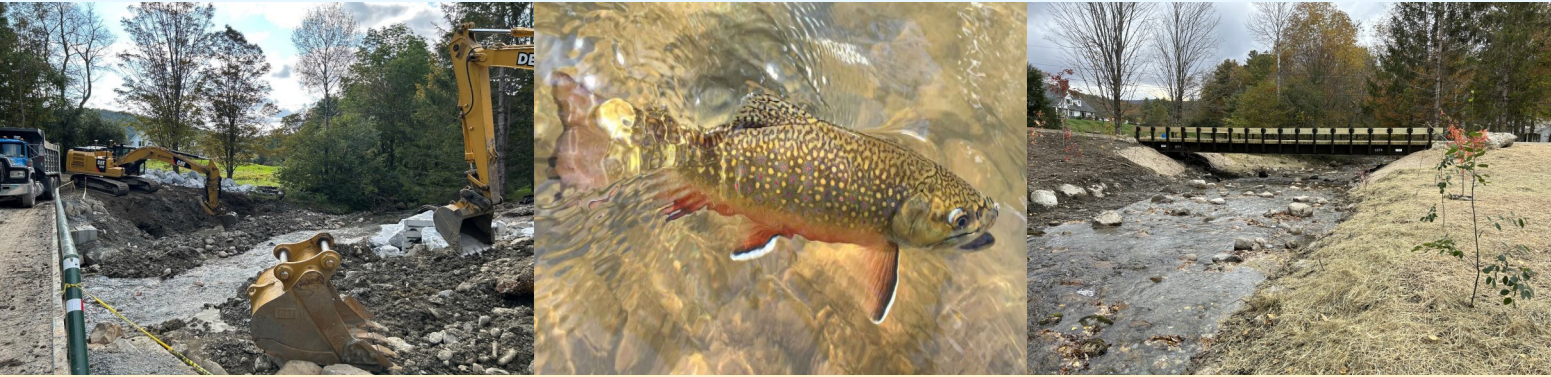
Davenport Excavation installs the new bridge abutments as the newly-undammed river flows through the project site.
