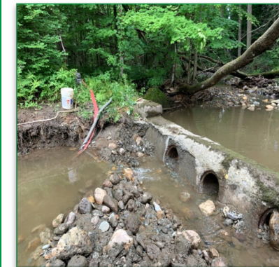
Davenport Excavation removes a dam on the Mettowee River.
