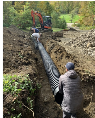
Andres Torizzo and Doug Tifft install a cross culvert.
